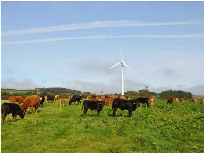
A 34m (Band B) turbine seen in front of a 20m (Band A) turbine at Carnebone Farm.
