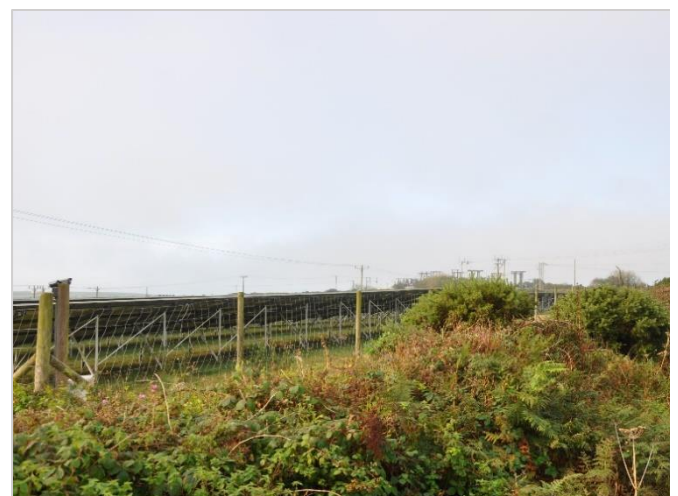
10ha (Band B) solar development at Nancrossa Farm seen in context of a substation.
