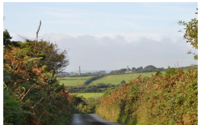
Engine houses punctuate the skyline (as seen from a lane lined with Cornish hedges).
