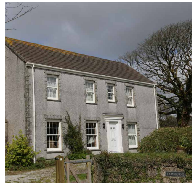
Figure 32: uPVC sash and one of few examples with flat concrete tiles.
