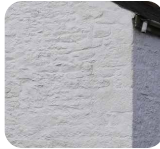
Lime washed rubble stone
