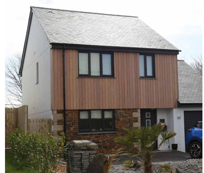
Figure 21: Smooth rendered gable, timber clad upper storey, contrasting stone façade lower storey and quoin. Dark uPVC.
