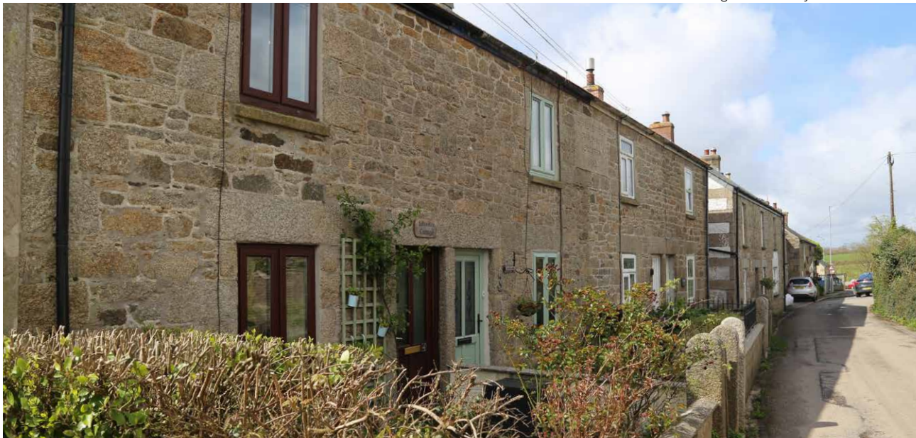
Figure 22: Traditional granite terrace, granite lintels and granite piers. Masonry boundary wall with coping
