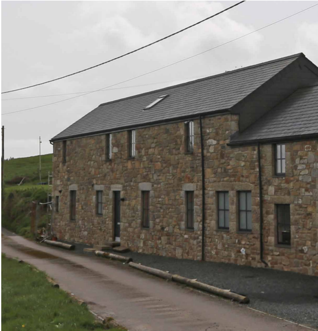
Figure 70: Renovated building demonstrates characteristic granite colours (cream, greys and buff) complimented by new slate roof and dark windows frames.
