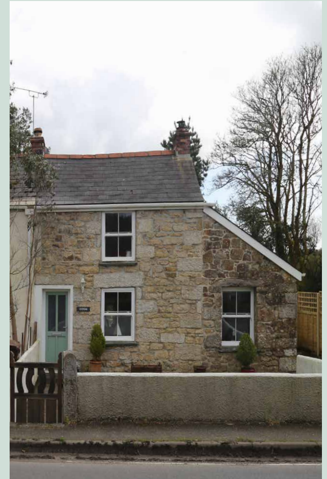
Figure 65: Simple stone cottage, uPVC sash and lean-to side extension. Characteristic very achievable precedent.
