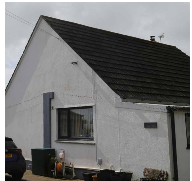
Figure 27: 45° concrete tile roof, heat pump.
