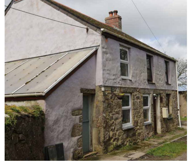
Figure 16: Depicted quoin, lower storey exposed stone and lean-to style extension.
