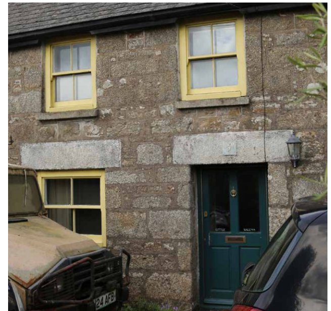
Figure 18: Exposed granite façade with large lintels. Timber sash windows.
