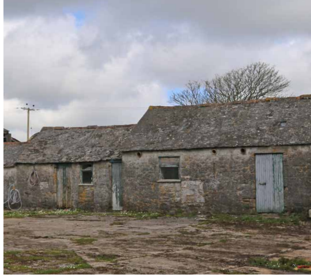
Figure 15: Staggered outbuilding roof, scantle tiles, vented terracotta ridge tiles.
