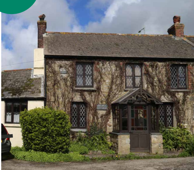
Figure 19: Stone façade, slate roof and sills. Dwarf wall porch, slate sill and coloured glazed lights.
