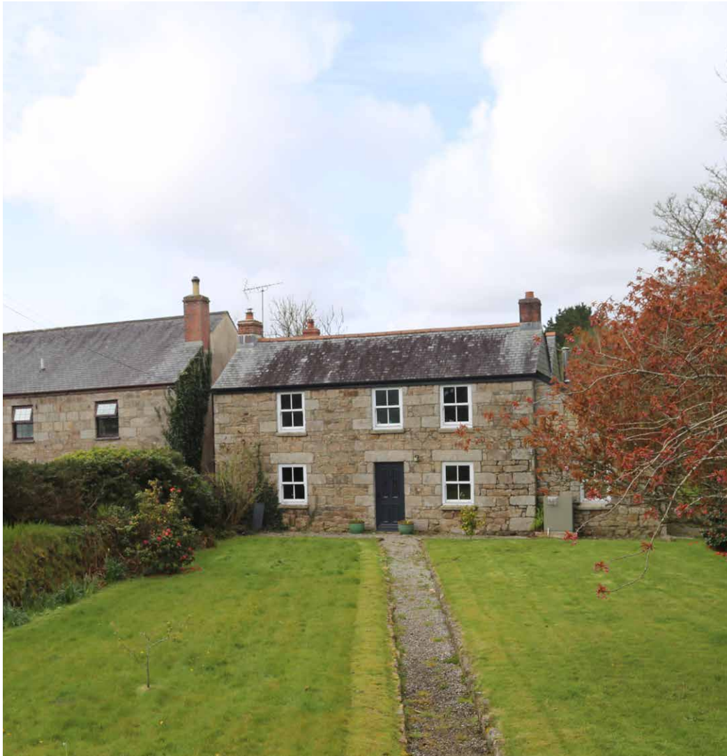
Figure 62: Simple long cottage with pitched slate roof, portrait balanced fenestration, and lean-to extension.
