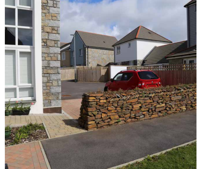
Figure 50: Parking courts at rear reduce car clutter at street level, however these fail to integrate green infrastructure (GI).
