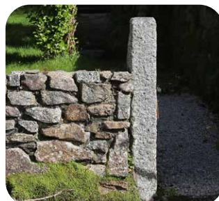
Granite gate piers
