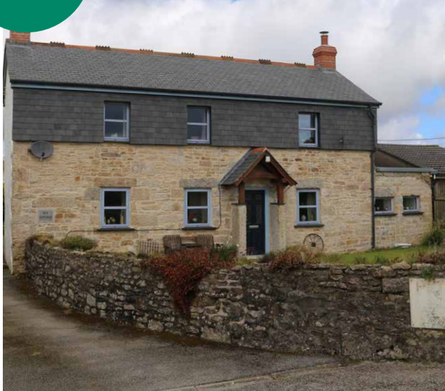
Figure 38: Upper storey slate hanging, granite façade with lime mortar.
