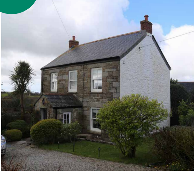
Figure 33: Pitched open fronted porch, granite façade .
