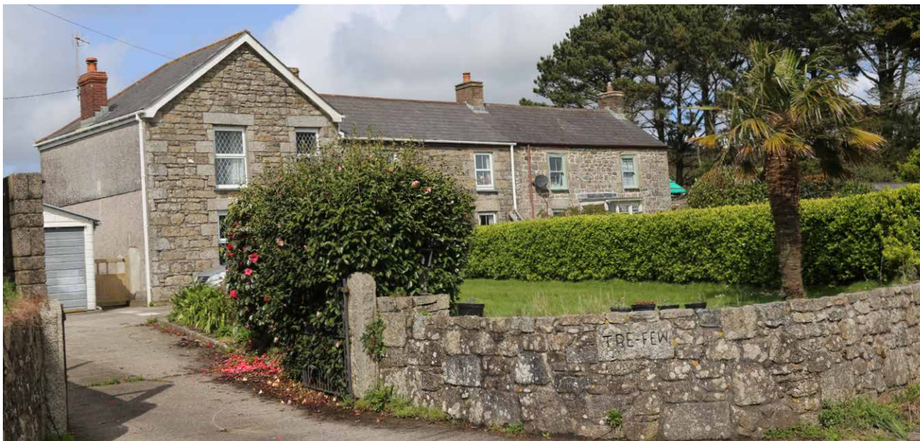
Figure 31: Crosswing configuration. Mortared stone boundary and façade, with contrasting stone detail.
