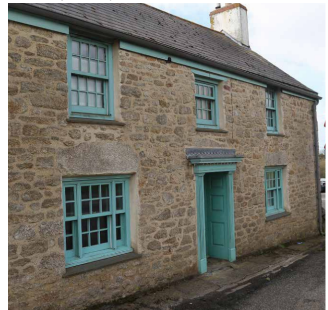
Figure 23: Craftsmanship demonstrated with windows and doors, including leadwork. Large granite lintels
