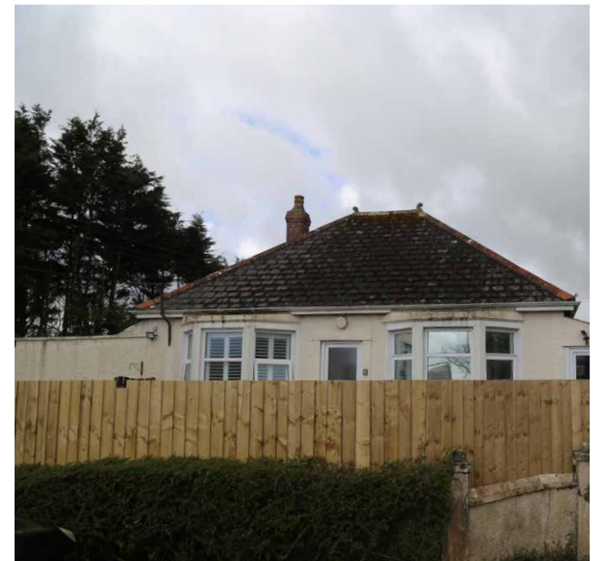
Figure 47: Poor quality fencing.
