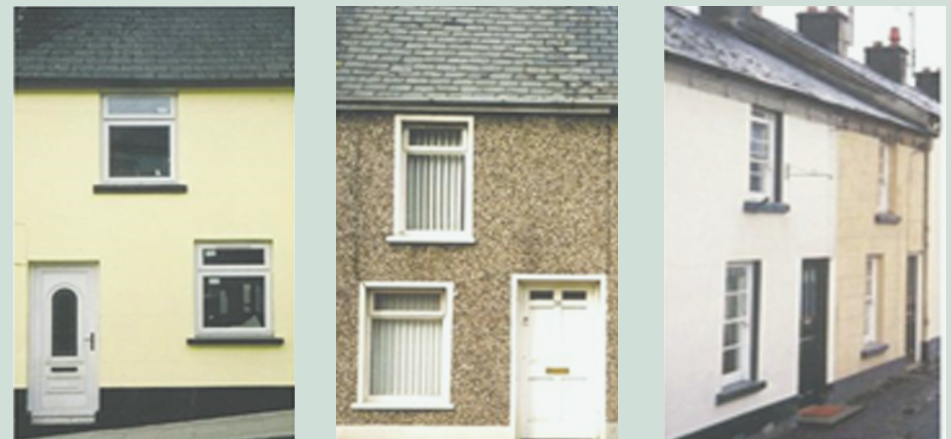
Figure 69: Example of original dwellings.
