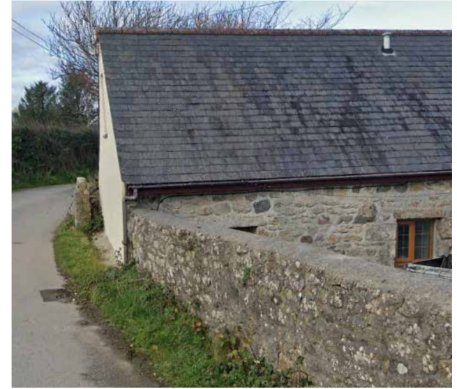
Figure 25: Building placed on boundary line. Rendered gable, exposed stone façade, stone wall contiguous and slate roof.
