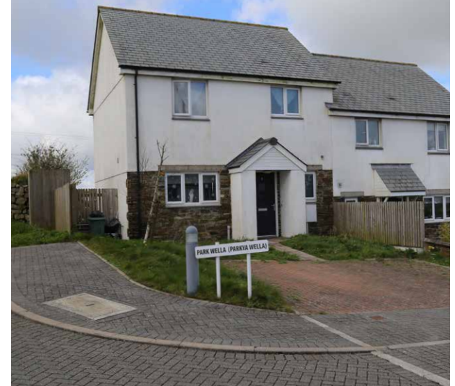
Figure 40: External surfaces and example of failed tree planting.
